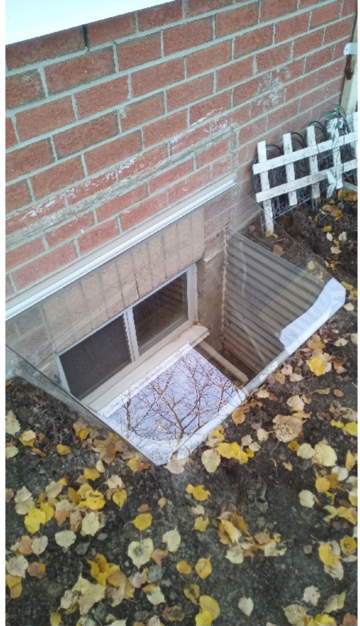
Cover in place
